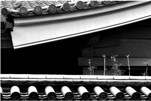
Jayne Marek, Winter Roofline , digital photograph, 2012.
